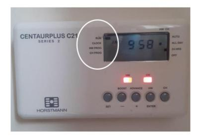
If there is no heat coming from the radiators, please make sure please make sure the red light is on at the CH point and that the on-radiator thermostat is not at '0', and the adjacent valve is turned all the way anti-clockwise:
